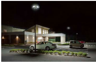
Example of Construction (Image)
